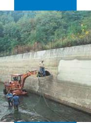
Application of Idrosilex Pronto by spray gun in hydroelectric canal
